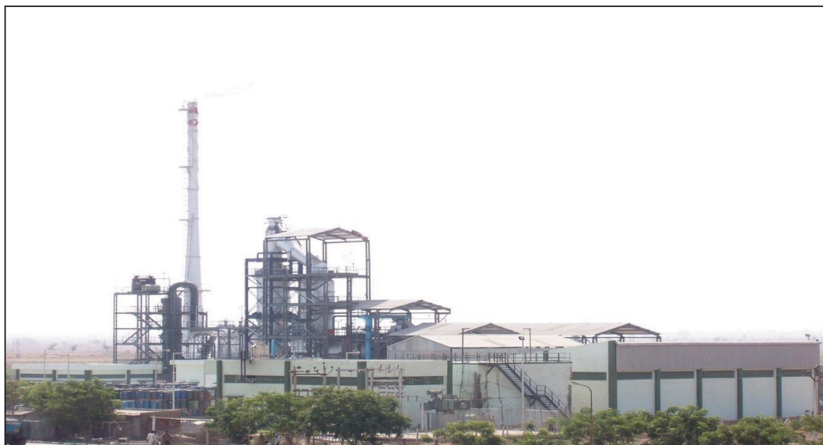
Figure: 9.1.1. Common Hazardous Waste Incinerator at Ankleshwar
