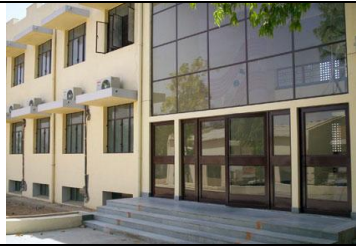
Main Building Side View
