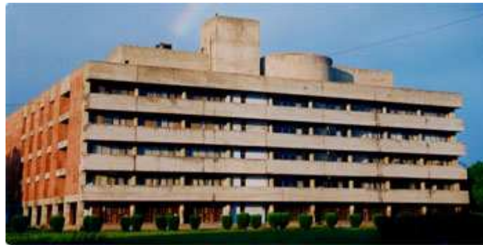
Figure 1: Panjab University Library Building
