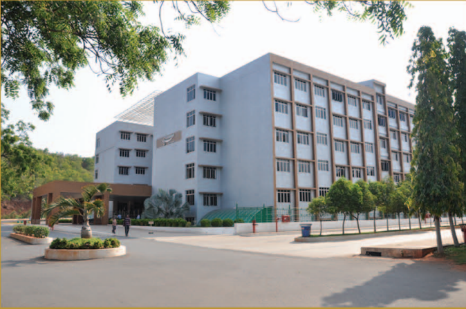
Chandras ICT Bhavan - Institute of Technology, Visakhapatnam Campus
