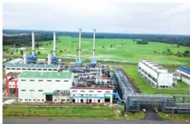
Captive Power Plant
