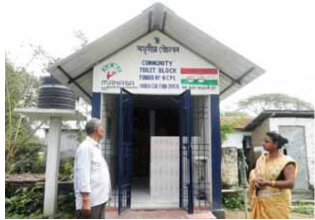
Community Sanitary Block & IHHL, Lakwa
