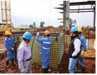
Ball Test for Air Preheater Tubes – 15MW Peat-to-power project at Gishoma
