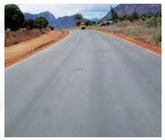
Laying of crushed stone base-G3 layer, Multinational Nacala Road Corridor Project
