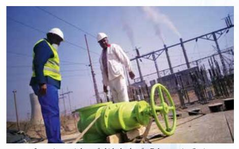
Inspection carried on refurbished valves for Deka pumping Station
