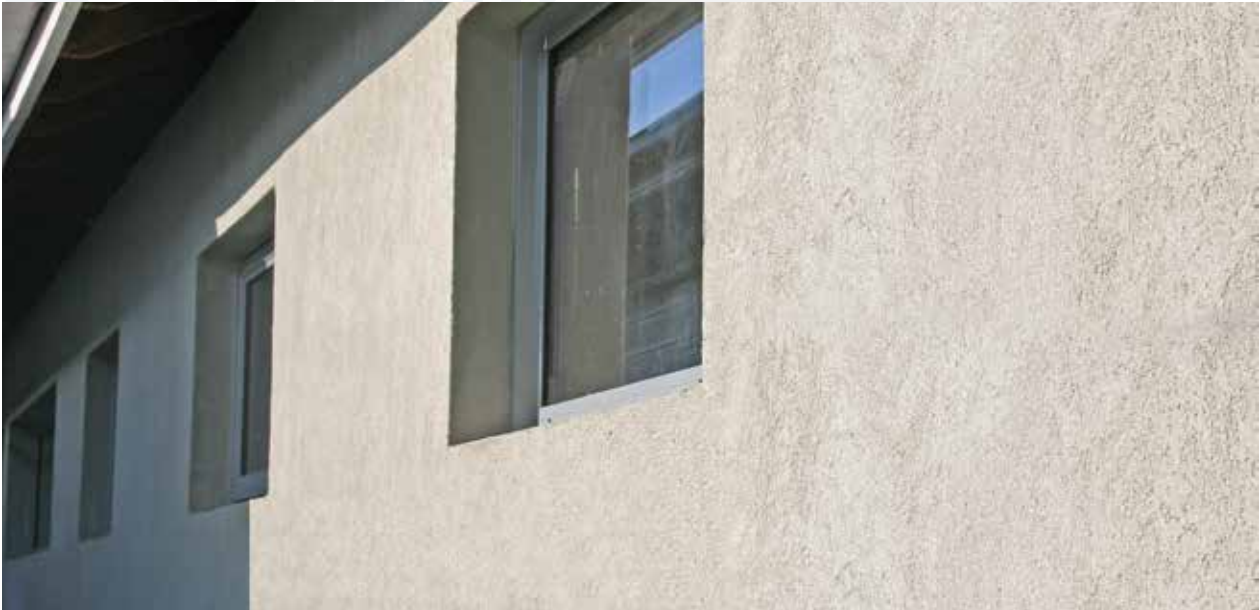
Photo 8. Complete RMAX Orange Board® render finished EIFS Cladded wall.
