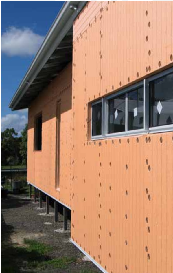
Photo 3. Installed RMAX Direct Fix EIFS EPS Grooved Cladding panels.
