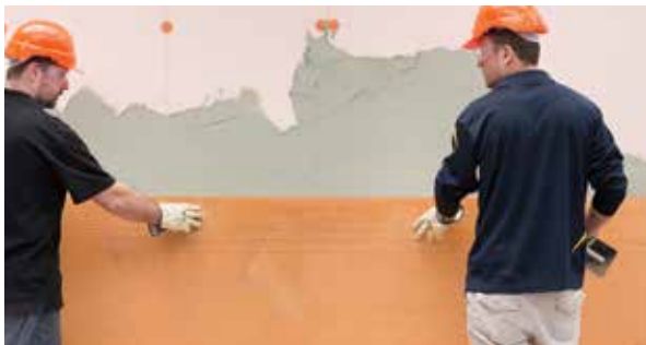
Photo 19. Application of Fibreglass Mesh over first render coat.
