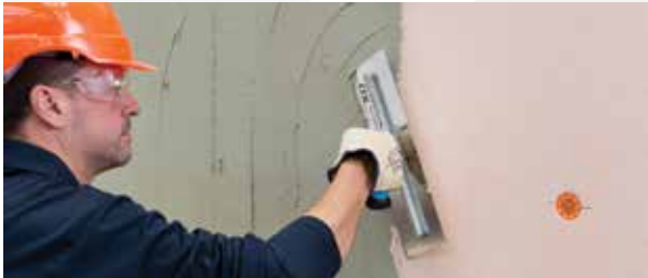
Photo 18. Application of first render coat.
