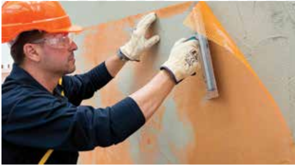
Photo 14. Embedding of Fibreglass Mesh into first render coat.
