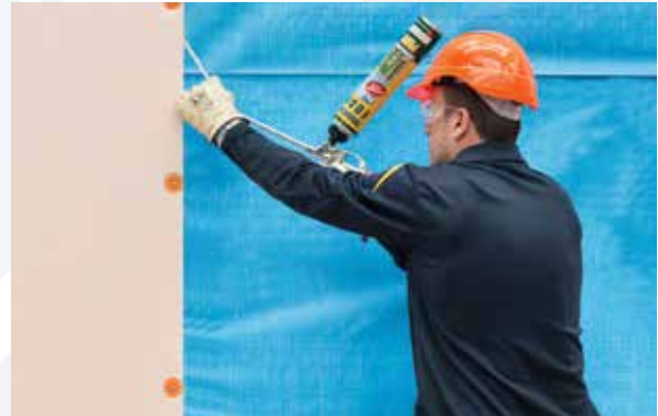
Photo 12. Adhesive Foam application to panel ends.
