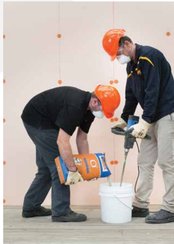
Photo 17. Preparation of Render Mix by addition of render and water.
