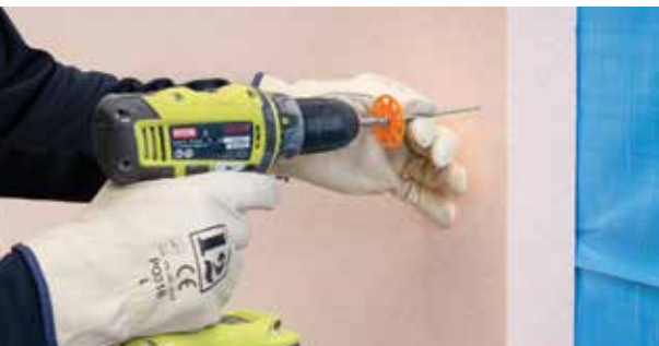
Photo 11. Installation of EIFS Cladding Panels directly to frame over Sarking.
