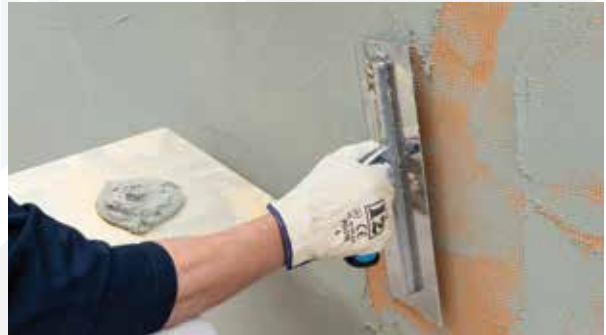
Photo 20. Embedding of Fibreglass Mesh into first render coat.
