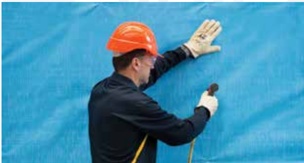
Photo 10. Installation of Sarking to frame.
