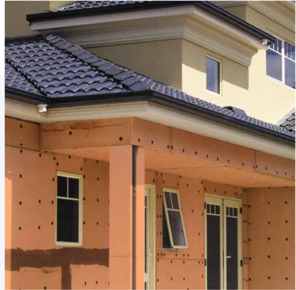
Photo 7. Top storey illustrates the finished rendered EIFS building facade whilst the bottom storey shows the standard RMAX EIFS Cladding Panels as installed directly to the stud frame.
