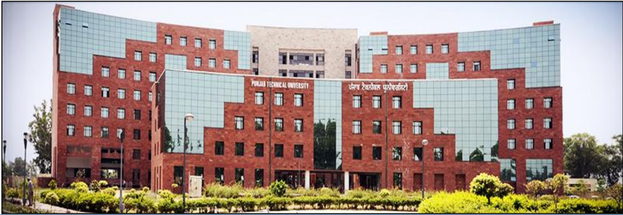
ADMINISTRATIVE BLOCK OF I. K. GUJRAL PUNJAB TECHNICAL UNIVERSITY, JALANDHAR
