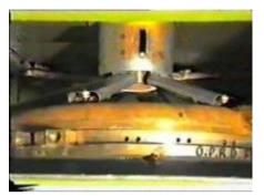
The Calandria Over Pressure Relief device (OPRD) is an 800-mm-diameter nozzle consisting of a stainless steel cover, which is held in position by shear pins. These pins break if the inside pressure in the calandria exceeds a pre-determined value of about 1.76 kg/cm<sup>2</sup><sub>(g)</sub>. To ensure a pressure-tight seal between the cover and the flanges, a
