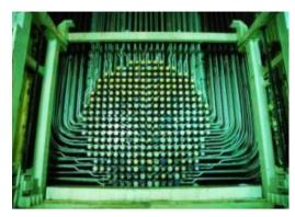
The feeders, made of carbon steel, are an important component of the primary heat transport (PHT) system in a PHWR. Feeder thinning on account of flow-assisted corrosion (FAC) was first noticed in 1995 in Candian PHWRs. The studies on FAC mechanism revealed that higher flow velocity at the bend portion of feeders along with the coolant pH of
