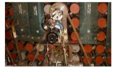
A light-water leak in O-10 channel of tri-junction weld joint between the calandria-side tube sheet, baffle plate and the lattice tube was detected and successfully repaired in Kaiga-3 south end-shield. The biggest challenge was to restrict the temperature of the nearby calandria tube rolling
