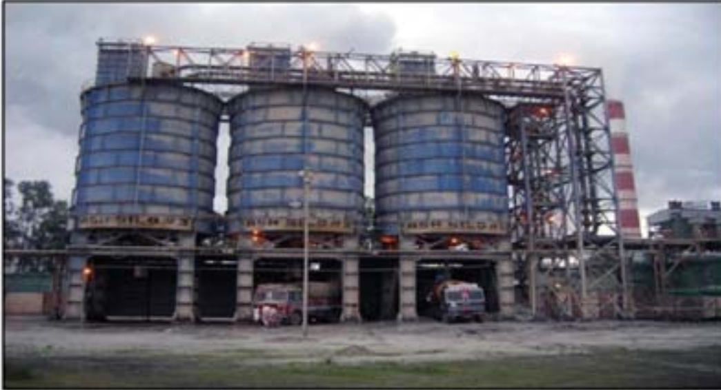
Figure 74: Dry Ash Disposal System
