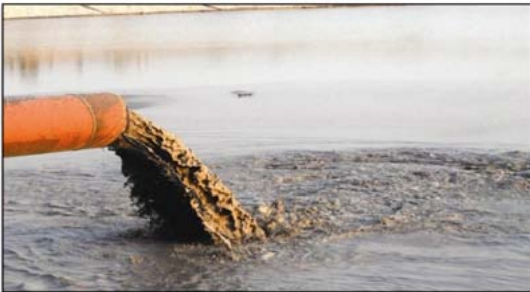
Figure 73: Wet Ash Disposal System
