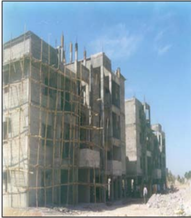
Figure 78: Building of Fly Ash Bricks
