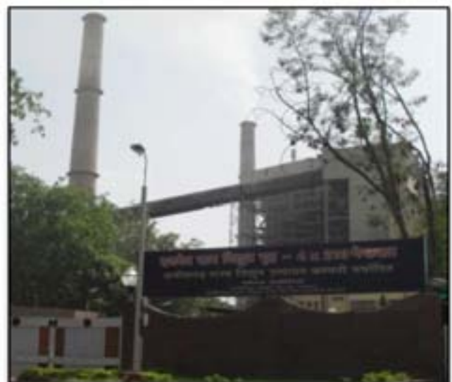
Figure 36 Hasdeo Thermal Power Station, Korba
