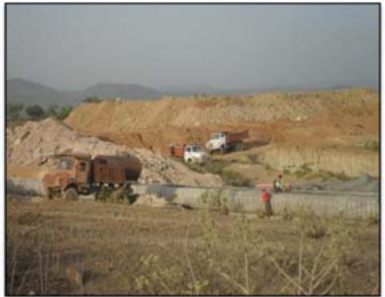
Figure 37: Ash dyke being developed for which HTPS has requested land diversion
