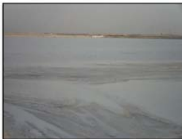
Figure 38 Ash dyke HTPS
