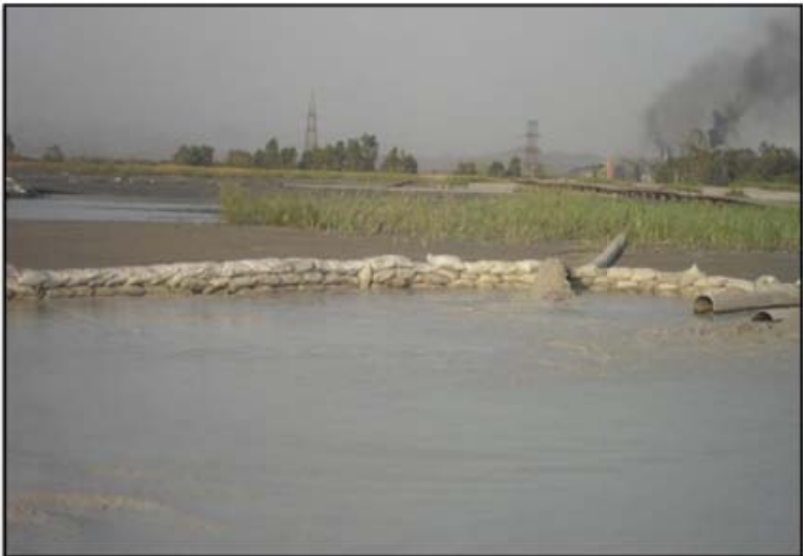
Figure 9 Power plant's ash dyke
