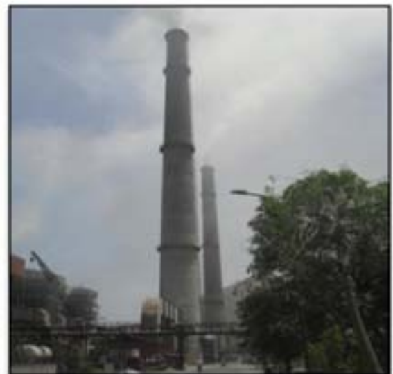
Figure 7 Satpura Power Station, Sarni
