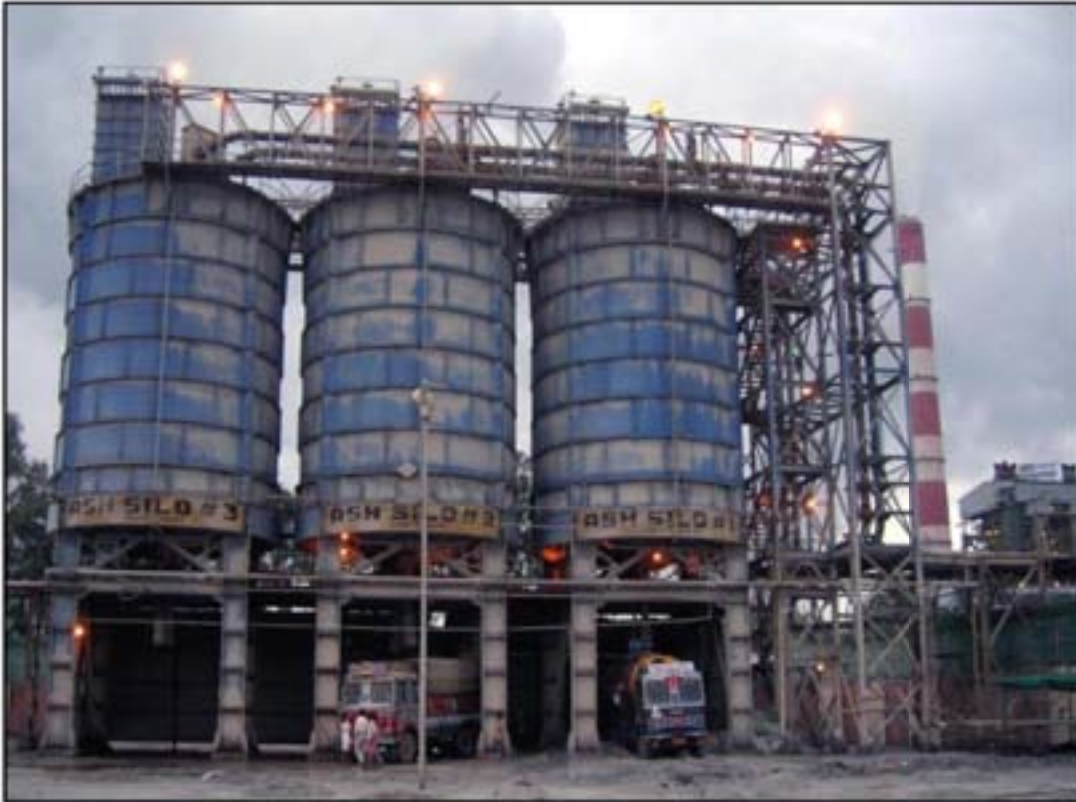
Figure 35 Ash silos, NTPC, Singrauli
