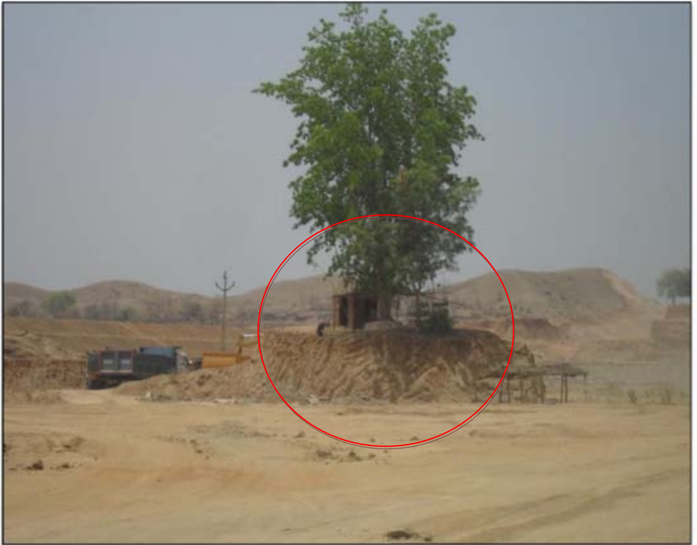
Figure 19 REL has changed plot maps to save trees that exist on the site area
