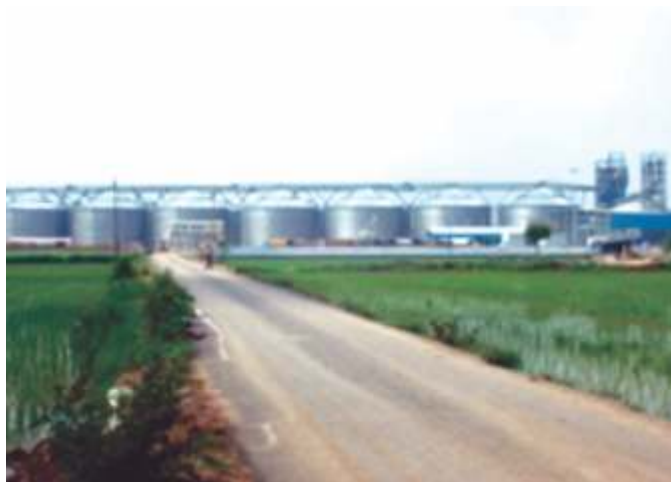
Silo storage facility for food grains at Moga
