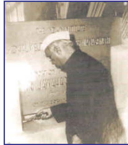
Pandit Jawaharlal Nehru laying the Foundation Stone of the Academic Block-1958
