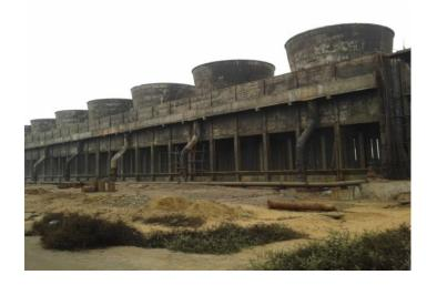
The hot water from condenser outlet reaches to cooling tower. Cooling towers are evaporative coolers to remove the heat of water so that water can be recirculating & can be reused. This heat of water is rejected to the atmosphere by evaporation. In NTPC modern types cooling tower uses in which cooling fan (suction) is required to remove the heat of water.
