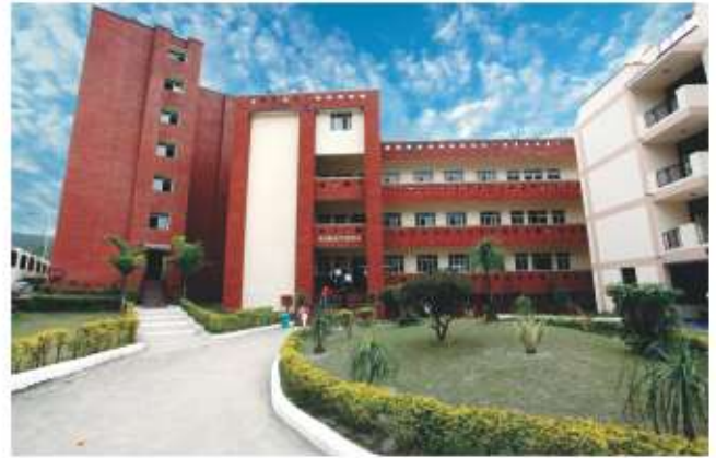
'Annapurna' - Multi-level Mess & Indoor Sports & Recreation Center
