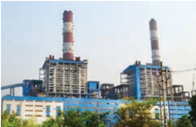
Indigenously manufactured supercritical set of 660 MW rating commissioned by BHEL at Barh 5
