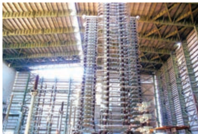
DC Hall, a pre-engineered building at HVDC Agra terminal, is an engineering landmark by BHEL in the field of HVDC Engineering
