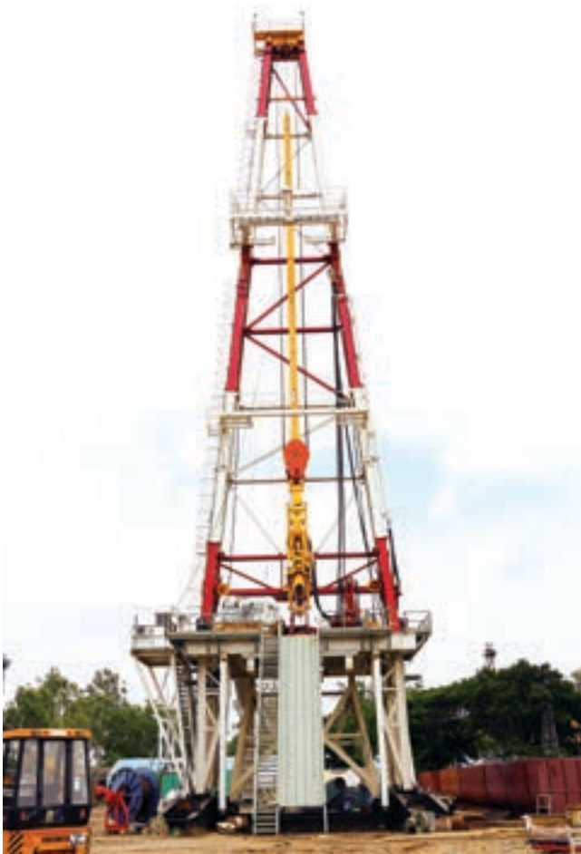
On-shore drilling rig with AC-SCR and AC-VFD technology
