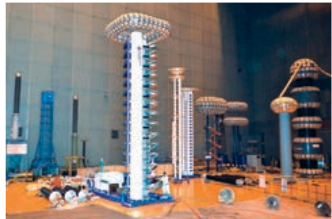
Series Resonant Tester with capability for testing of 1200 kV class power transformers installed at HEP, Bhopal
