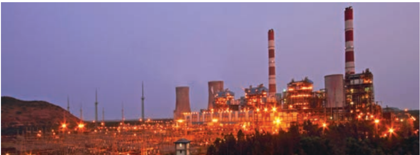
4x500 MW Simhadri STPS commissioned by BHEL
