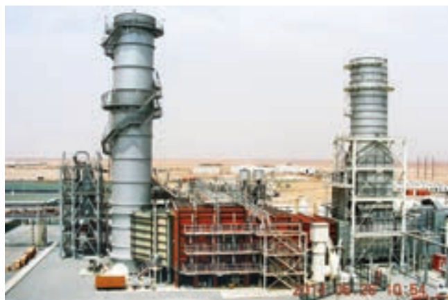
126 MW Qarn Alam-3 Power Project executed by BHEL at Oman
