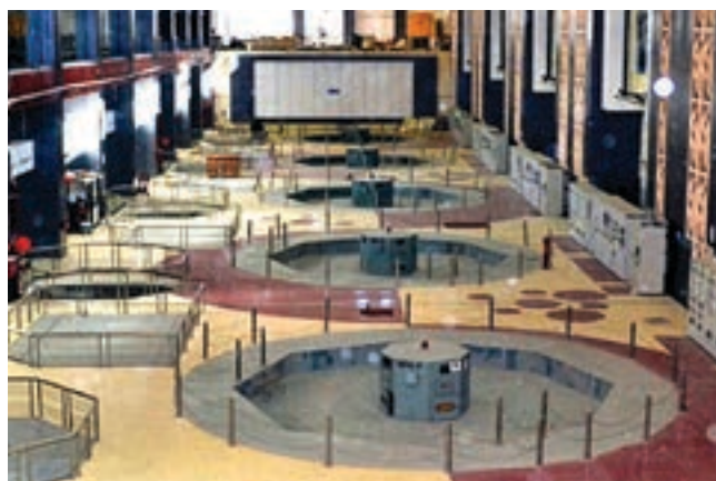
Rampur Hydro Electric Project awarded National Gold Award for Early Completion (2013-14)
