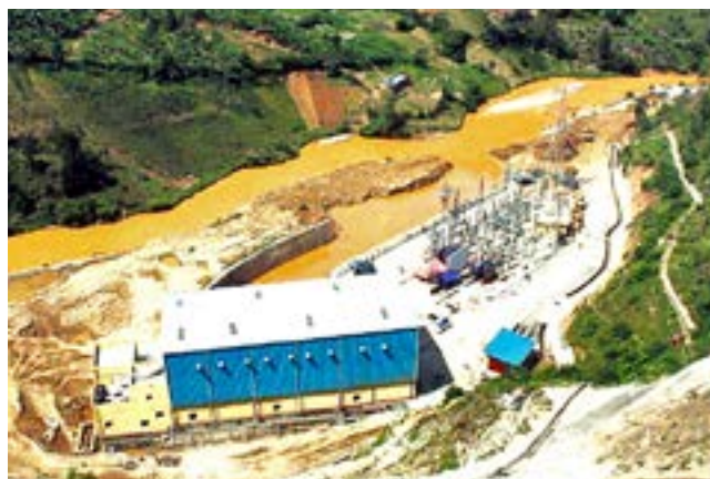
2x14 MW Nyabarongo Hydro Electric Project commissioned by BHEL in Rwanda
