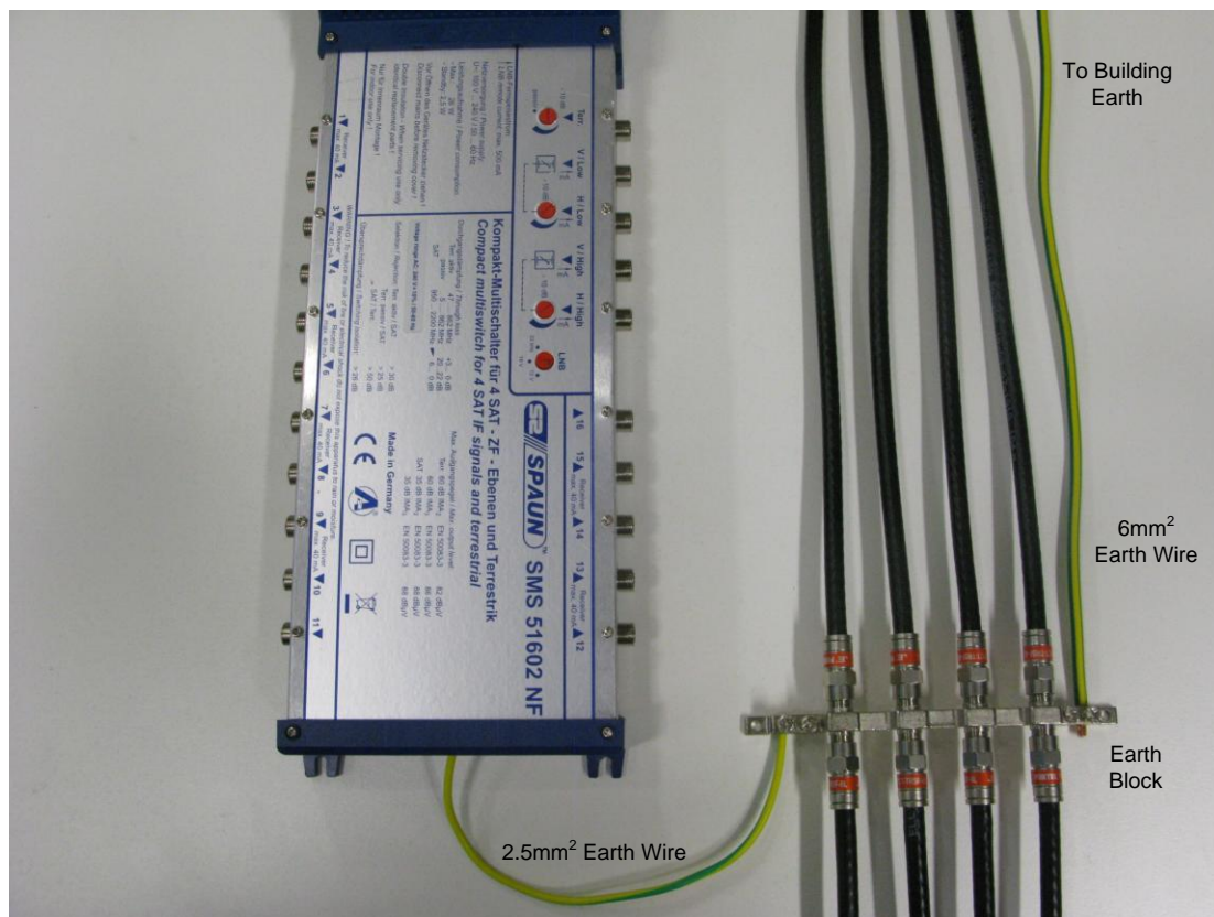
Figure 23 – Earthing Example – Passive Method
