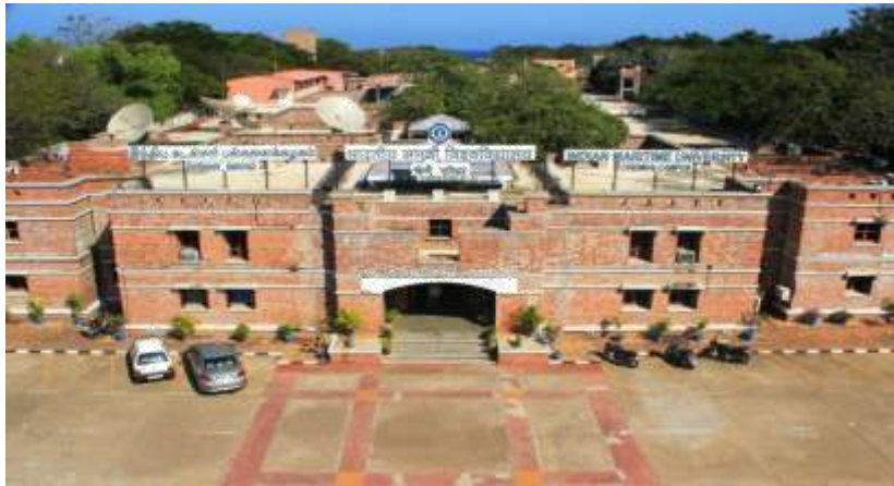
Aerial View of IMU, Chennai Campus
