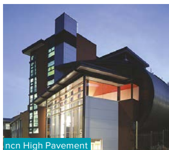
ncn High Pavement
