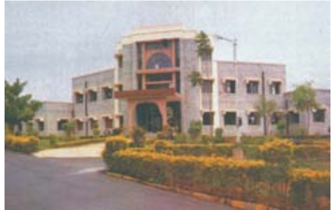
Hot Line Training Centre, Bengaluru
