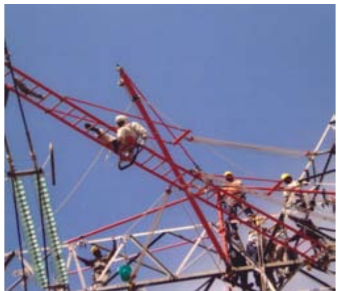
Hot Line Maintenance Techniques at HLTC, Bengaluru
