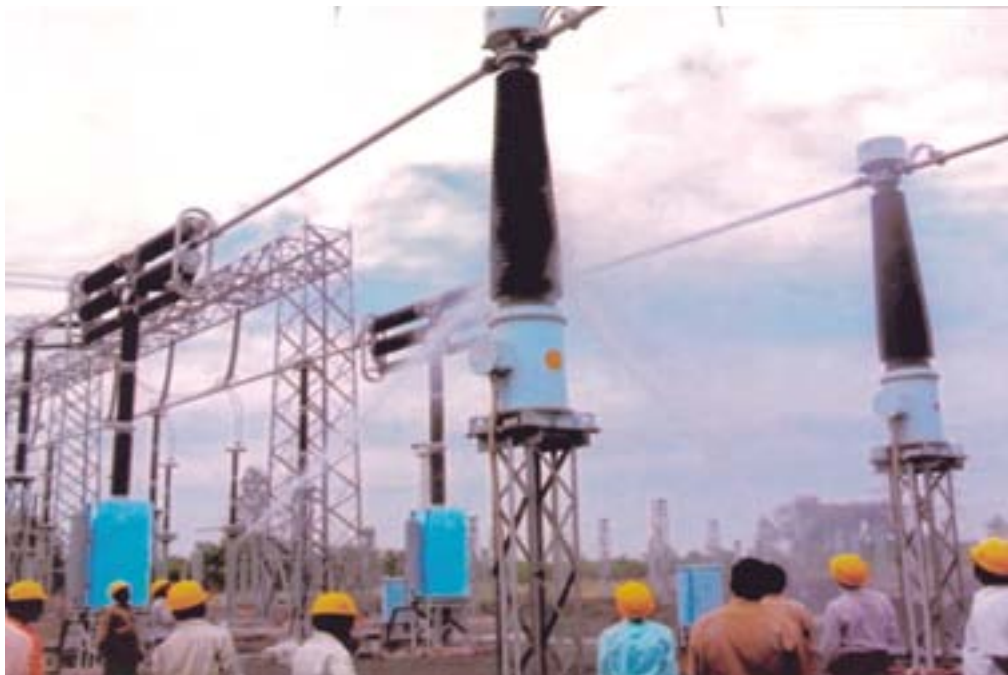
Live Line Insulator Washing Techniques, HLTC, Bengaluru
