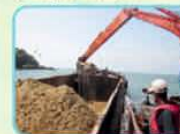
Field visit on soil investigation
